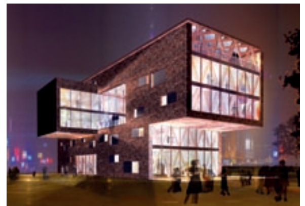
Hamburg House in Shanghai
